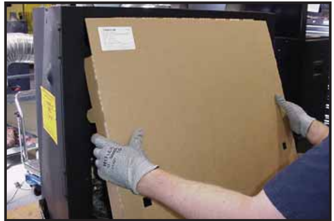
Figure 13.4 Installation of Splatter Guard
